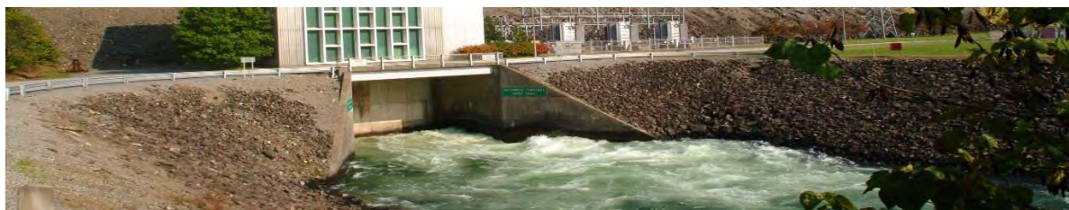
Figure 3.6. Weir Structure at South Holston Dam
