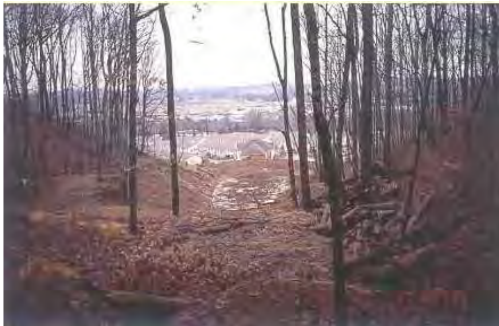
Figure 3.41. 2003 Forest Ridge Apartments Landslide
