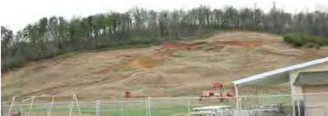
Figure 3.40. 2003 Forest Ridge Apartments Landslide
